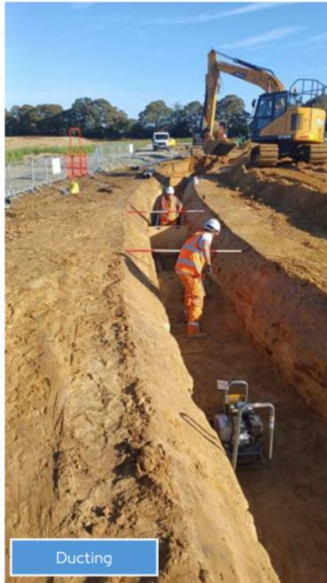
Figure 2: Orsted Hornsea 3 –onshore HVDC cable duct excavation 8
